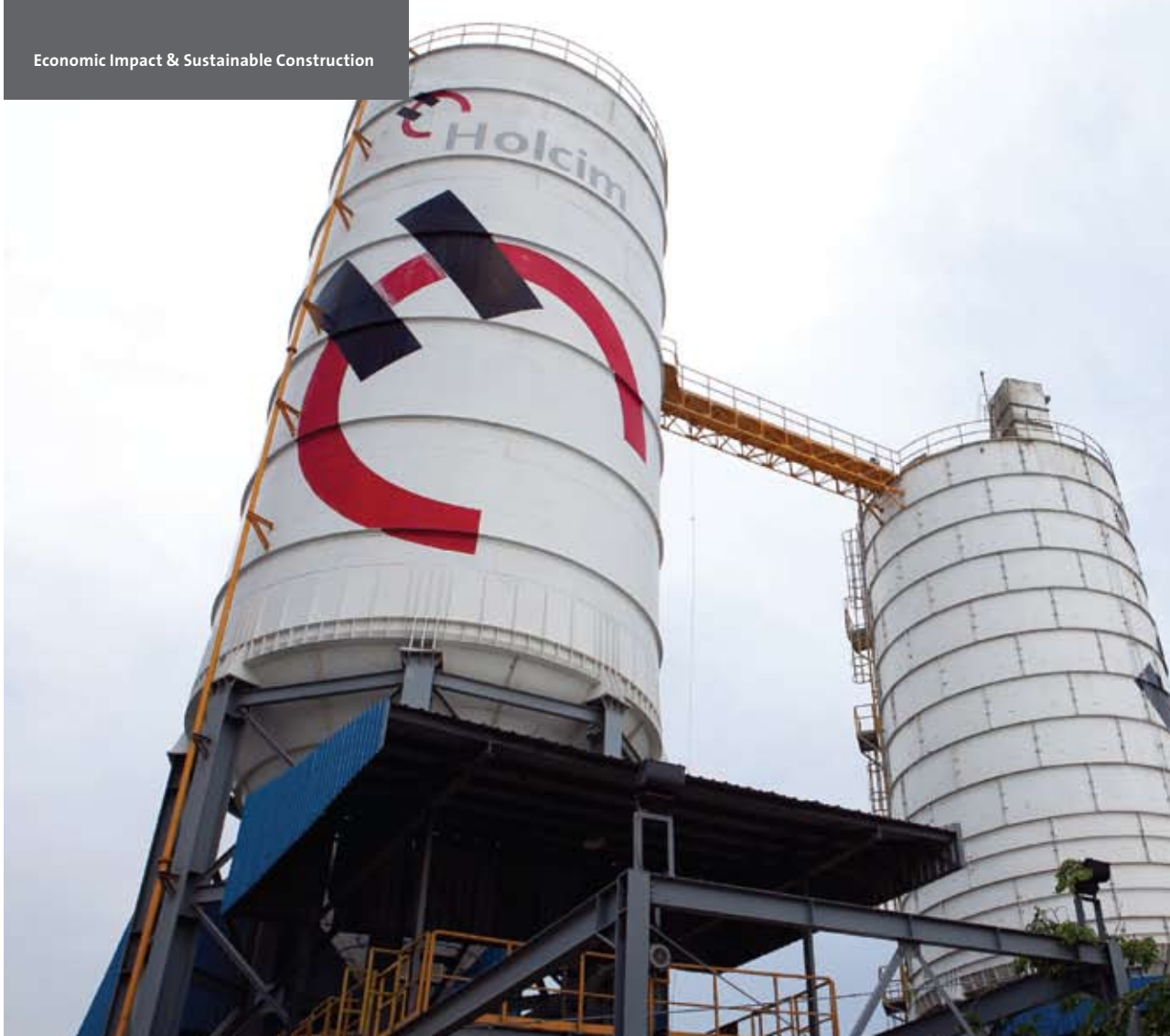
Holcim silos, Romokalisari, Surabaya. During 2012 we revamped out logistics.
