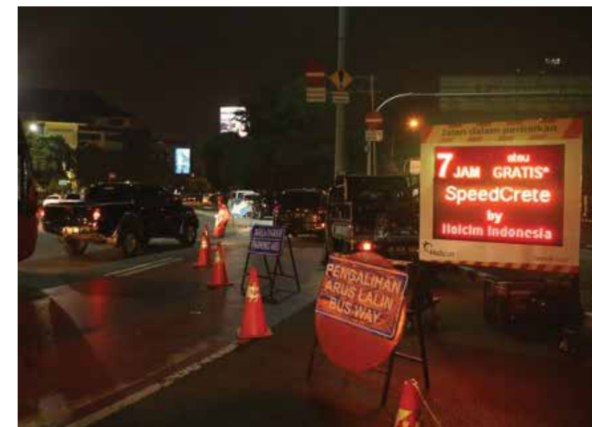
Overnight road repairs, in just seven hours.
