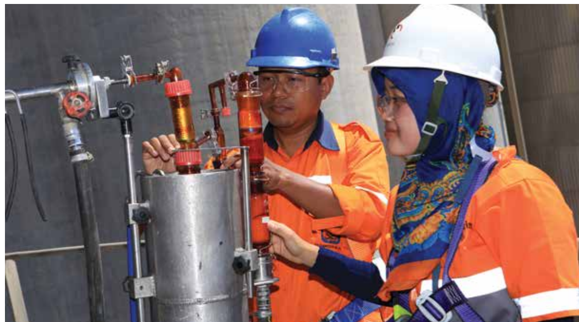
Emissions are monitored regularly to ensure regulatory requirements are met.
