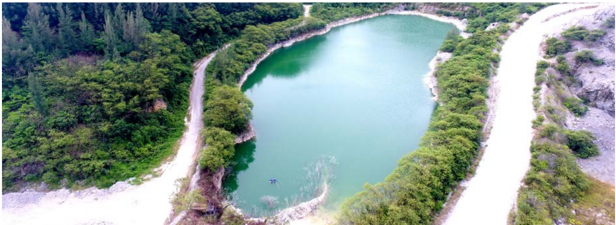
Fasilitas pemanfaatan air hujan Pabrik Lhoknga. Lhoknga Plant rainwater utilization facility.
