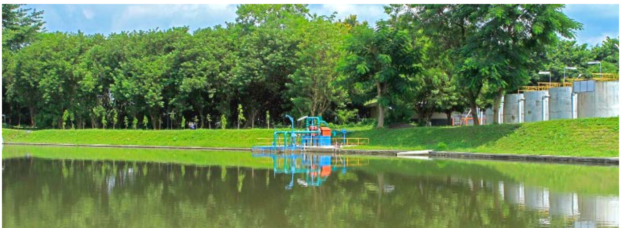
Fasilitas pemanfaatan air hujan Pabrik Cilacap. Cilacap Plant rainwater utilization facility.
