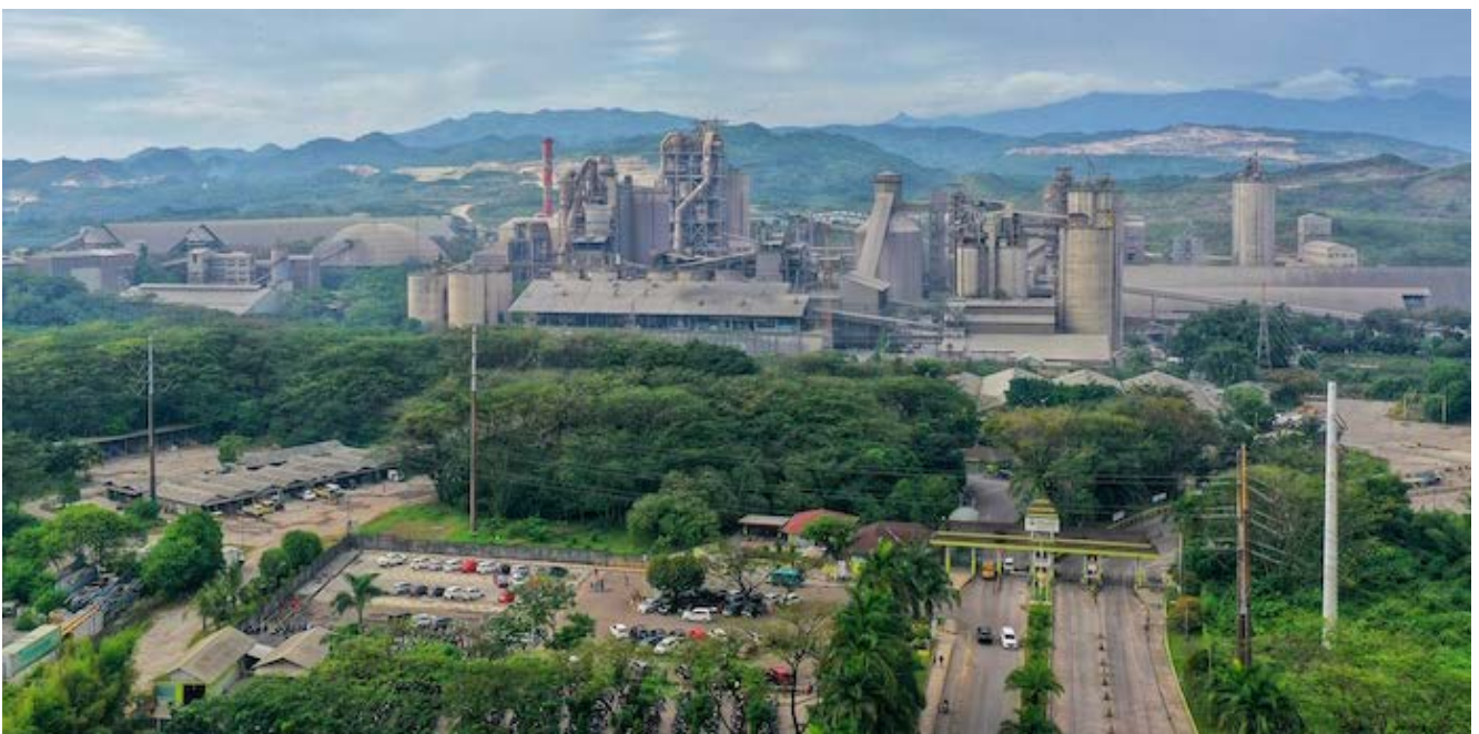
Pabrik Narogong, Jawa Barat. Narogong Plant, West Java.
